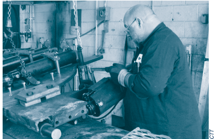
Paul Zuck, maintenance mechanic at Jackson CRC, uses a hydraulic bottle jack to replace a spring that is part of the height adjustment system for an underbody scraper that he is rebuilding.
