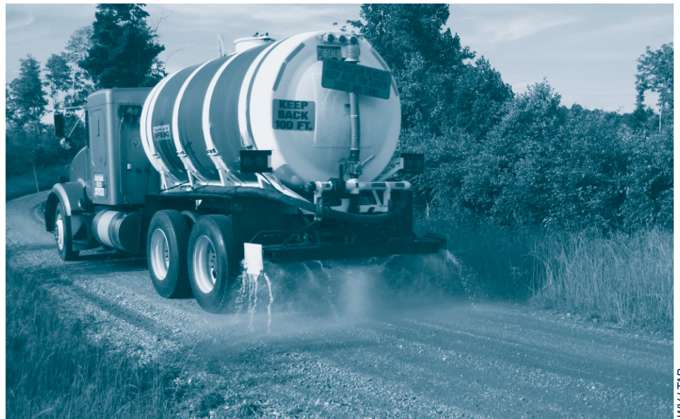
A tanker truck applied five different dust control materials to gravel roads for the project. Calcium chloride was the most effective of the materials tested.
