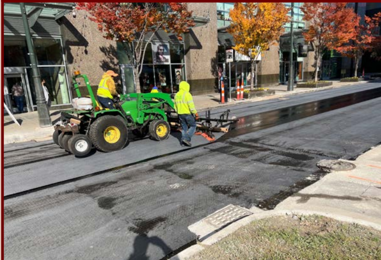
Repaving Monroe Street, Detroit, with composite paving grid. Top left: Rolls of 12.5-foot-wide Mirafi MPG4 fabric. Top right: Cutting the composite paving grid fabric to size. Bottom left: Placing the fabric. Bottom right: Paving over the fabric with asphalt. (Photo: Courtesy of City of Detroit)
