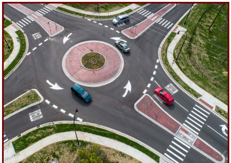
Compact roundabout in Washtenaw County designed by MacDonell (Photo: Courtesy of Washtenaw CRC)
