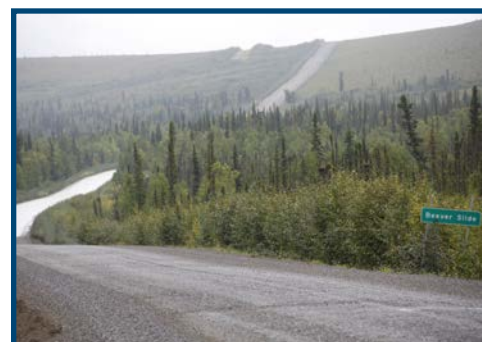
Beaver Slide before wicking fabric installed (Photo: Courtesy of Solmax)
