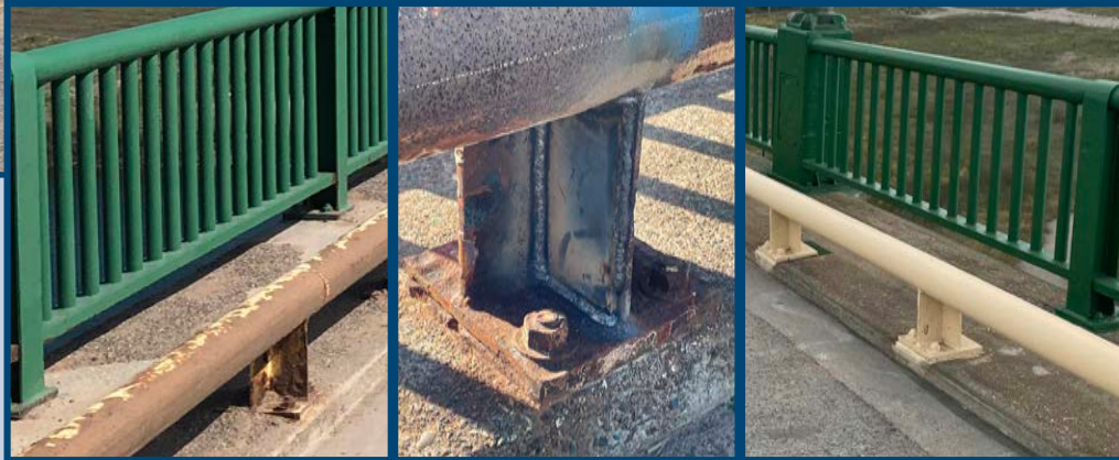
Pedestrian and curb rail painted with HRCSA on east (right) side and not painted on west (left) side.
