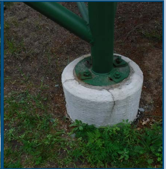
Stair support system (left) and base (right) of pedestrian bridge over US-31 in Traverse City painted with HRCSA as seen in 2021 inspection report (Photos: Courtesy of MDOT)
