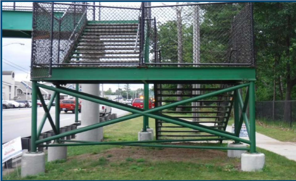
Stair support system (left) and base (right) of pedestrian bridge over US-31 in Traverse City painted with HRCSA as seen in 2021 inspection report (Photos: Courtesy of MDOT)
