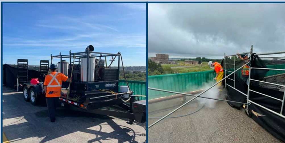
Left: Pressure washer; Right: Pressure washing the curb rail (Photos: Courtesy of IBA)
