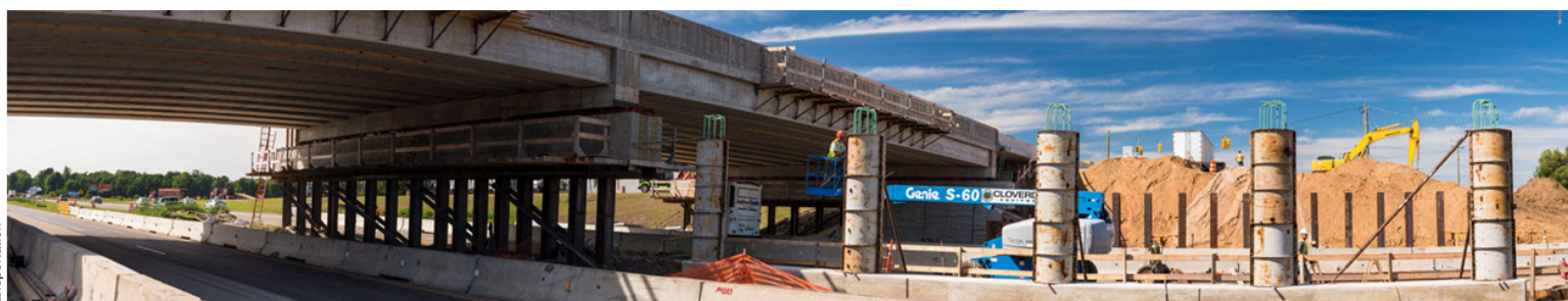
Innovative M-50 or I-96 bridge slide by the Michigan Department of Transportation
