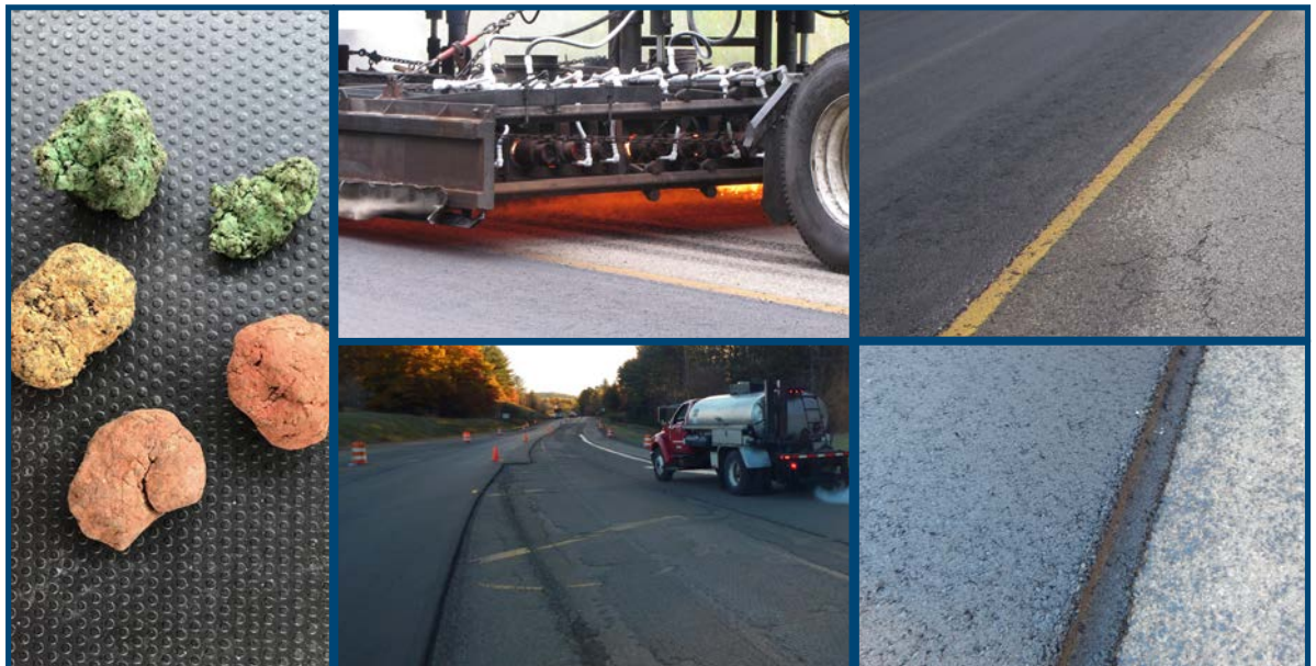
Left: Asphalt pellets, originally grey, are now colored to show the performance grade of the asphalt. Right top (two photos): Dickinson CRC hot in-place recycled asphalt paving project in 2016. Right bottom (two photos): Dickinson CRC fiber-reinforced asphalt paving project in 2020. (Photos courtesy of Dickinson CRC).
