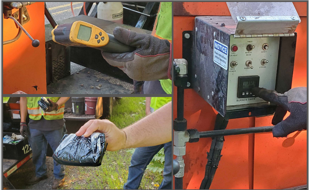
Steps in using a trailer-mounted asphalt recycler: (counterclockwise from right) setting the burner timer, checking the temperature of the mix with a gun, adding rejuvenator pucks (Photos: CTT Archive).
