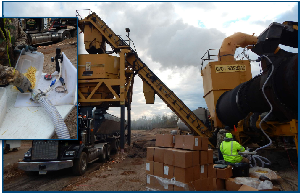
Feeding aramid fibers into the asphalt (Photos: Courtesy of Dickinson CRC)
