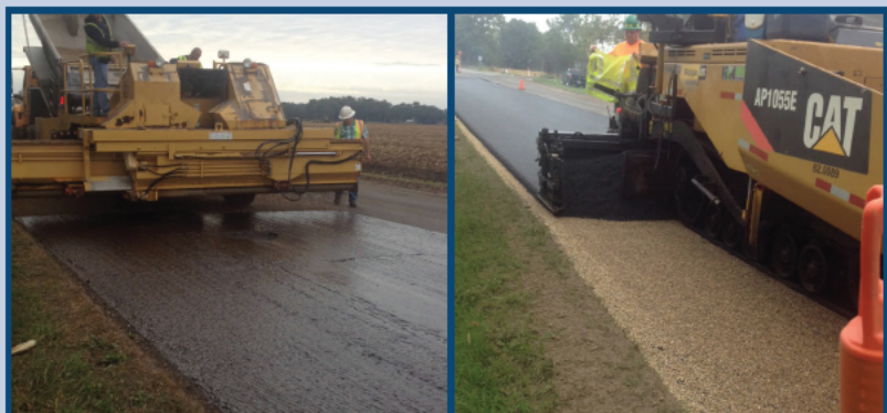
A Texas underseal on Kalamazoo County's Portage Road: spreading aggregate for the chip seal (left) and paving with an HMA over the chip seal (right)
