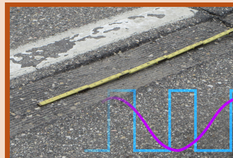
Mumble strips’ sine-wave-like cut in pavement 2 ; overlay shows profile of rumble strips (blue line) versus mumble strips (purple line). 4
