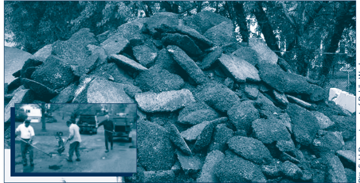
The City of Pittsfield's stockpile of cured blacktop cookies. Inset photo: Pittsfield maintenance crew filling potholes with reheated blacktop cookies.
