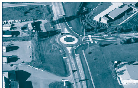
A roundabout, completed in July 2006 in Otsego County, Michigan, drastically reduced congestion and crashes at a busy rural intersection.
