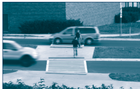
A channelized median provides a pedestrian refuge area to help students cross US-41 on the campus of Michigan Technological University in Houghton.
