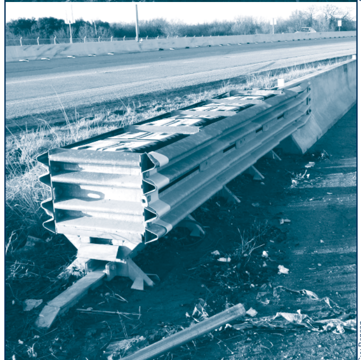
Breakaway traffic sign and what remains of a crash cushion the author's car hit after skidding off the road one morning.
